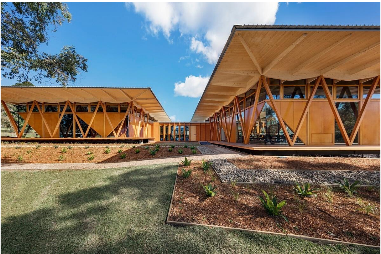
IRON ASH treated MASSLAM 45 V-Columns at Macquarie University, 'Incubator', NSW, Australia.
