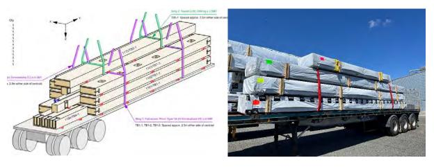
ATC panels arrive on site in trucks ready to lift in reverse installation sequence according to approved loading plans. Panels are accompanied by a set of marking plans highlighting their position within the build, assembly drawings to see the connection details, and individual shop drawings to nominate lifting and weight of panels.
