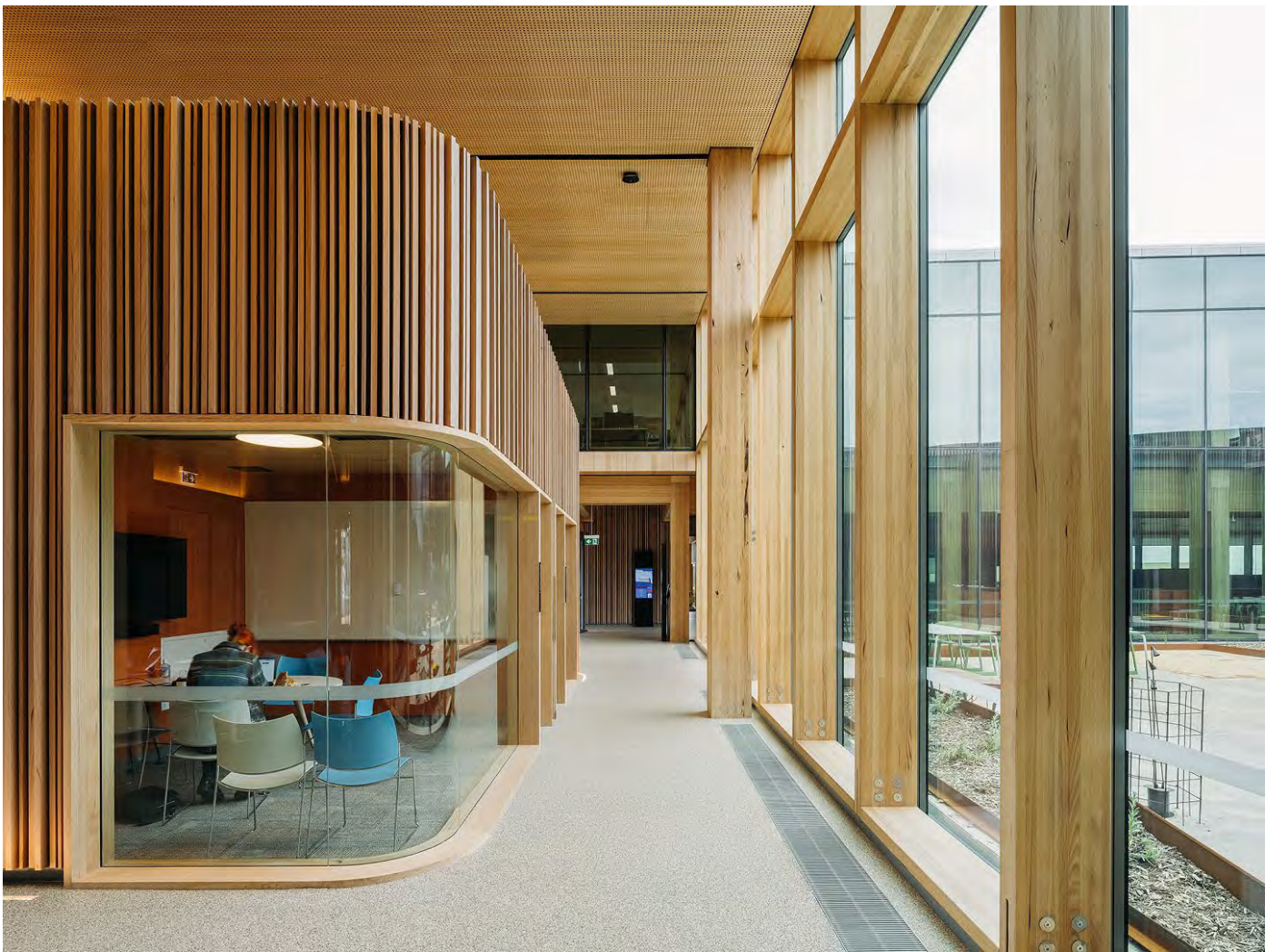
MASSLAM 45 columns at the University of Tasmania, Burnie, Australia.
